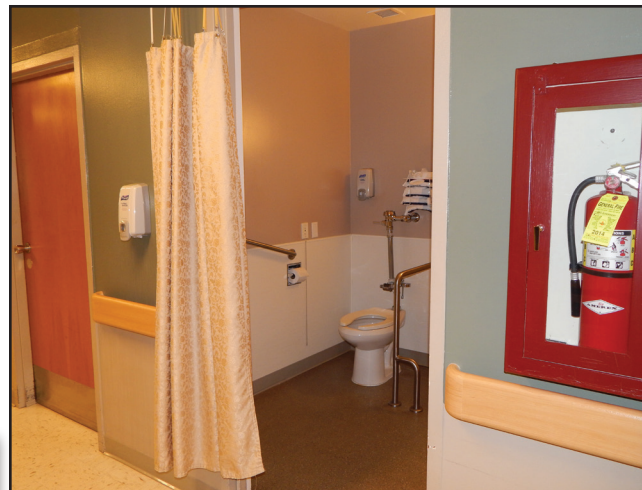
Existing Layout: Nursing Home Shared Hallway Restroom
